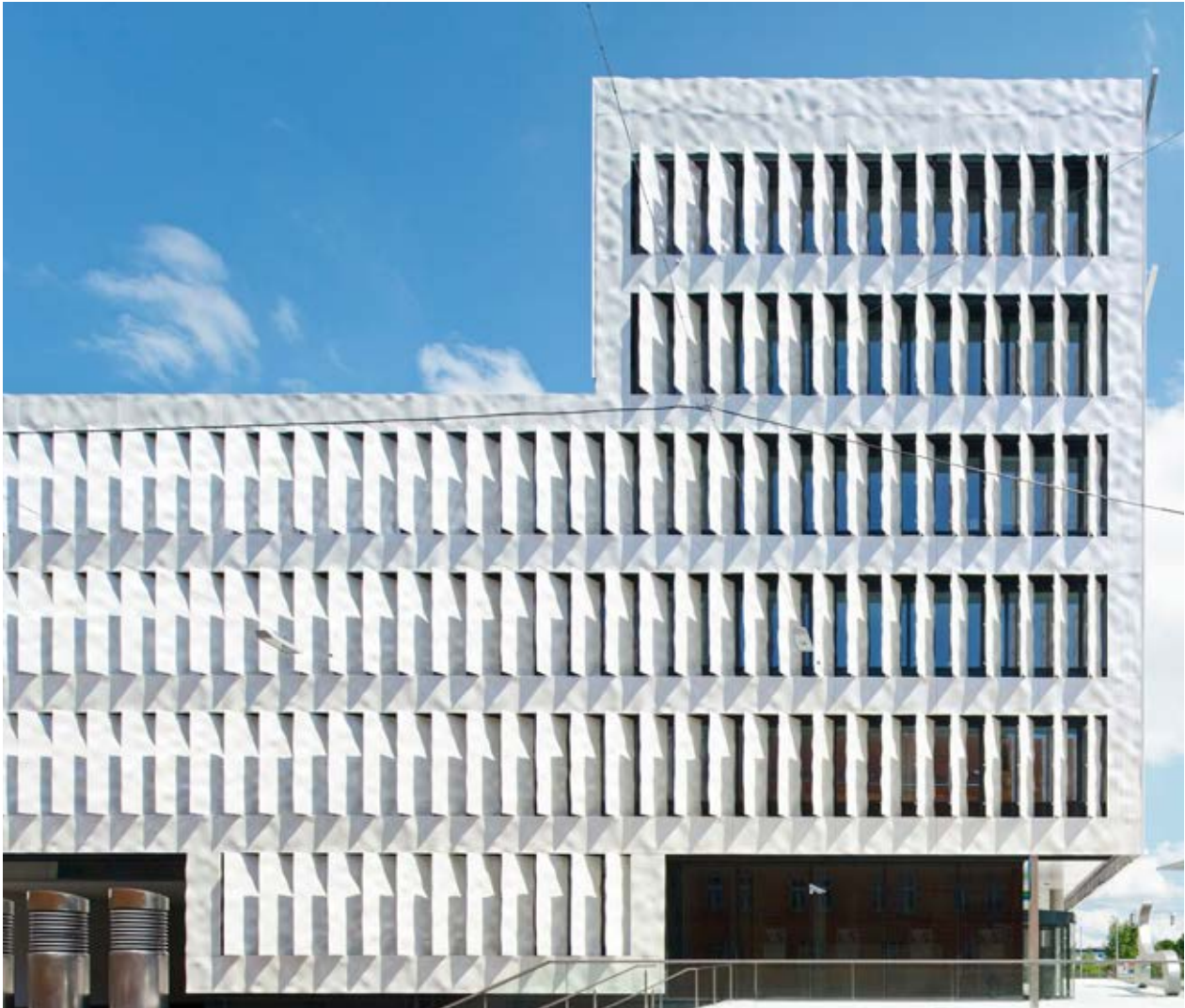
HYPO NOE GROUP ARCHITECTURE PRODUCT PHOTO ST. POELTEN, AUSTRIA ZIESER ZT LTD. SPECIAL - 3D PLATE "DUNE ST. POELTEN", ALUMINIUM, DURAFLON® COATING RUPERT STEINER
